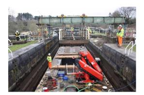
The renovation work involves cleaning, shot-blasting and priming to prevent further corrosion, before the bridge is put into storage for 12 months. The second phase of the renovation works, depending on available funds, would be in spring 2017 and include extensive repairs and re-painting of the structure.
