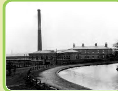
A pumping station to transfer brine to Runcorn stood next to the cottages, close to the canal bridge.
